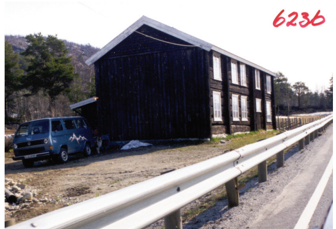
Large, solid massive wooden house along the E-136 in Lesja, Norway. It's impossible to tell the sound insulation just by inspection, measurements are essential to make the right decision. The figure 6236 is a tag number. Results are not available at the time of printing.
