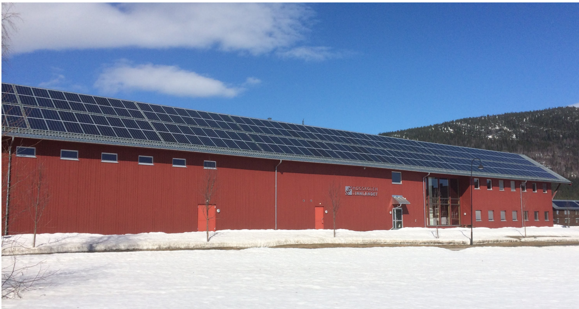
FIGURE 5.4: South-faced roof-mounted PV system at Campus Evenstad.
