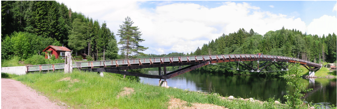
Figure 8.14 Lardal pedestrian bridge
