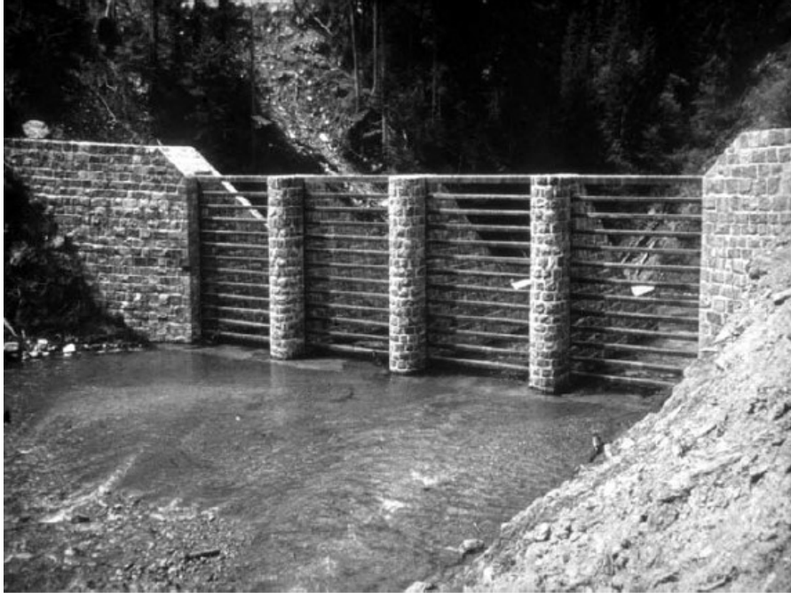
Figure 2-9: Sectional barrier with fins/beams in Maerzenbach, Tyrol, Austria (Hübl et al., 2005)
