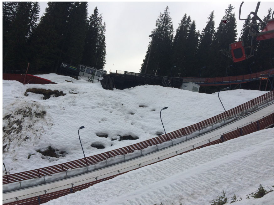
Figure A.4: Light poles in conjunction with jump stadium, which has not been included in the calculations
