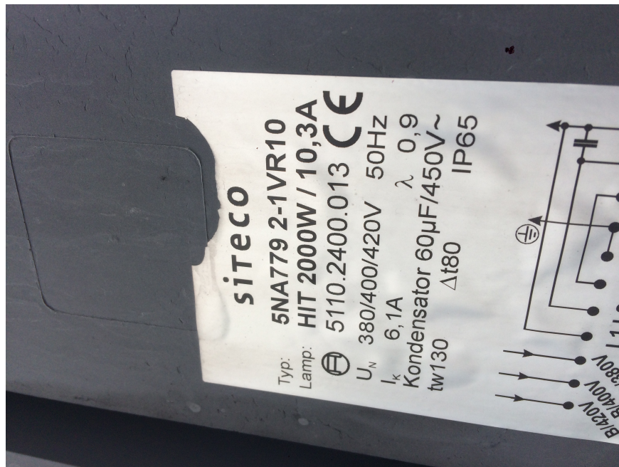
Figure A.2: Power ratings of lights in Granåsen
