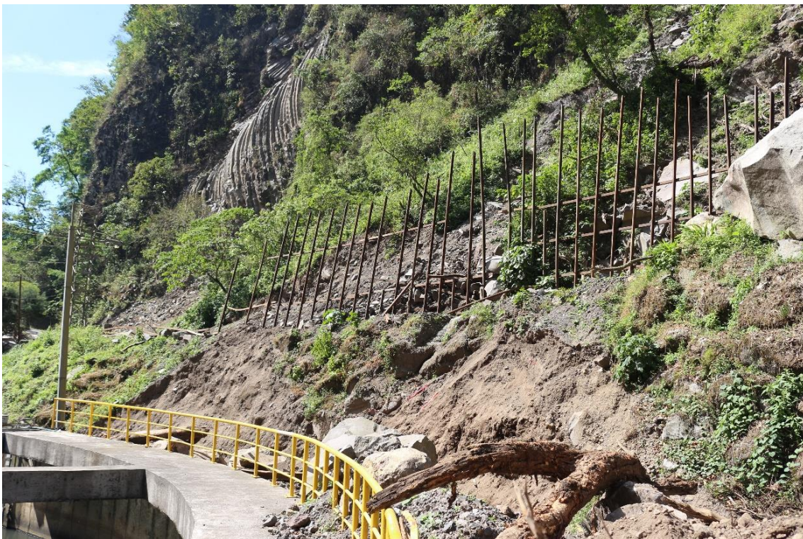
Figure 4.1 Landslide throwing sediments to El Canadá HPP Headworks.
