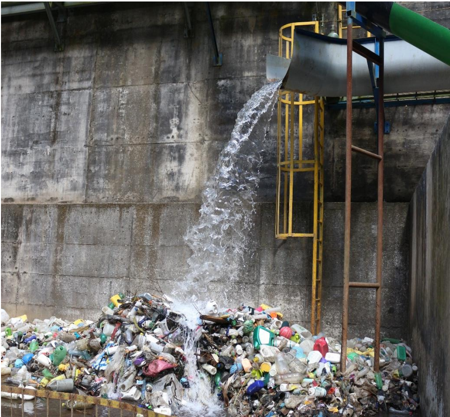
Figure 5.4 Disposal area for collecting garbage and debris.
