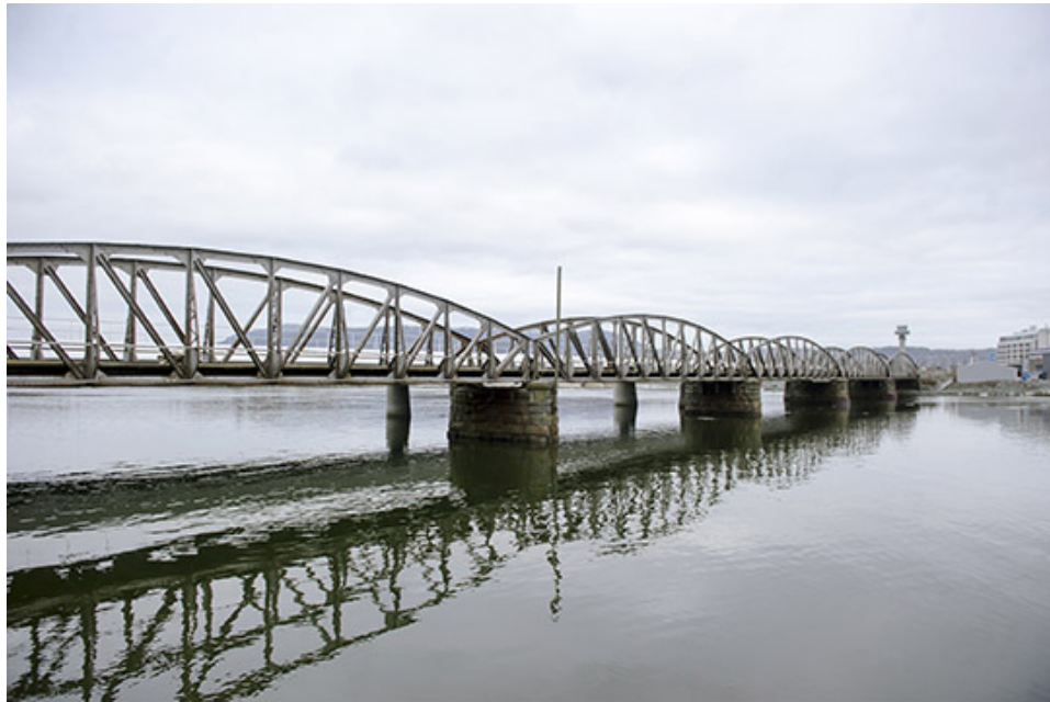
Figure 3.1: Hell Bridge when still in normal service.
