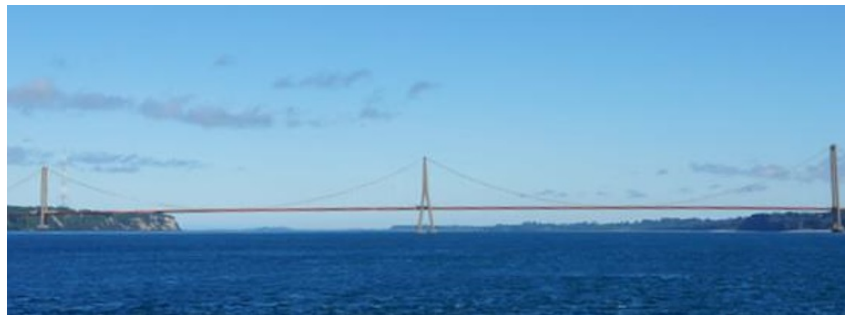
Figure 2.3: Picture of multi-span suspension bridge Chacao Bridge. [KAA, 2016]
