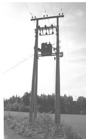
Figure 3 Pole-mounted transformer arrangement
