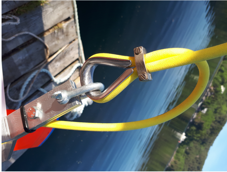
Figure 4.19: Mounting of cable
