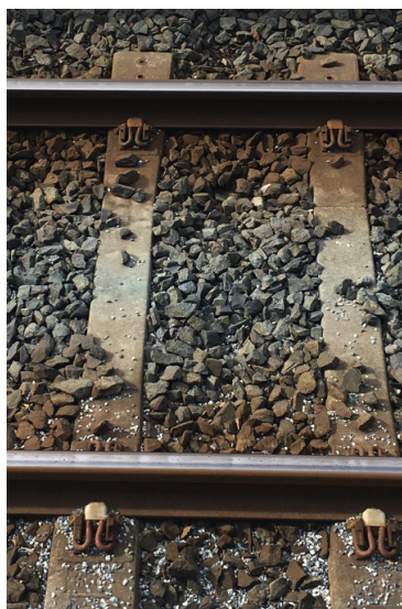
Figure 3.2: Part of 49E1 rail track with JBV 97 sleeper and gravel base.
