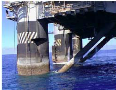
Figure 1: Column leg after supply vessel impact (Do Amaral Amante et al., 2008)
