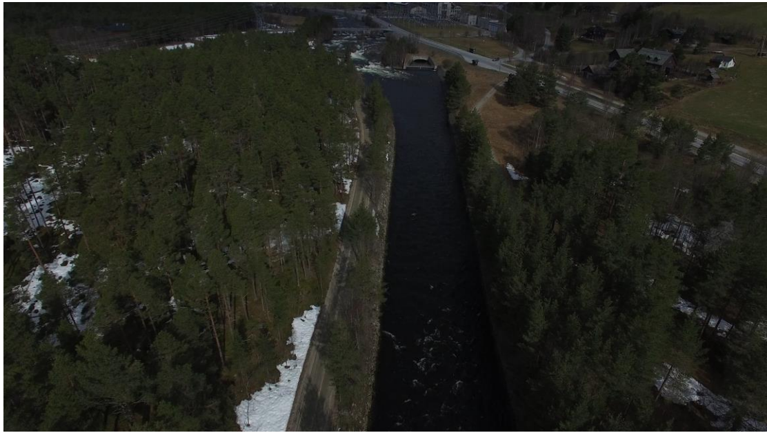
Figure G1. Outlet and channel
