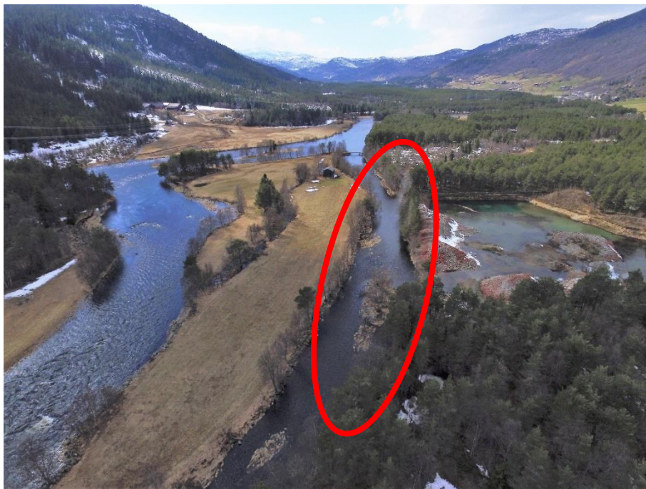
Figure G5. Gjerdeøyne from downstream. Indicated the northern stream in Gjerdeøyne, as potential location to take mitigation measurements.
