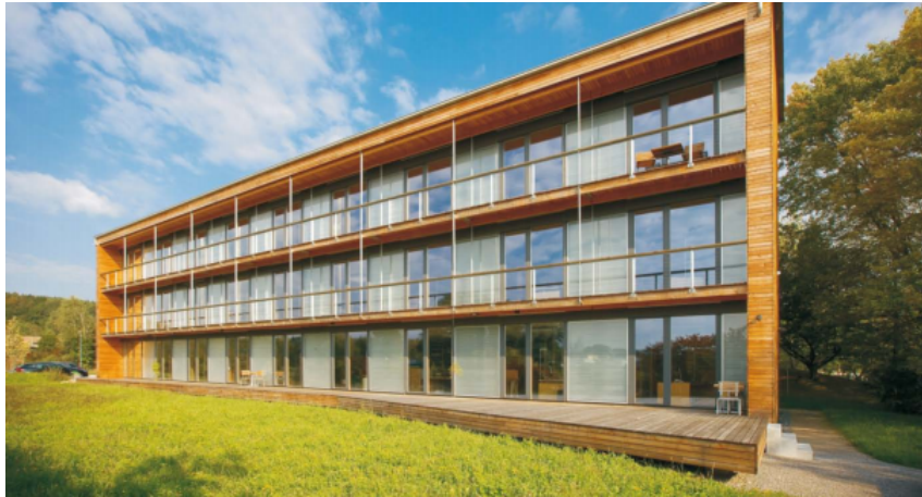
Figure 1.24: Image of an office building in Zurich with PCM in the windows (GLASSX AG, n.d.[a])
