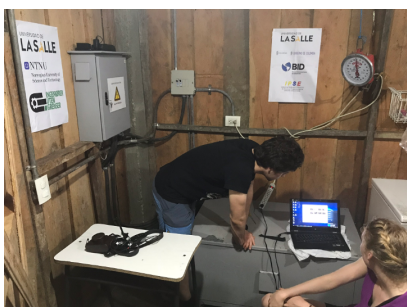
Fig. 4. Installation Process in the refrigeration center
