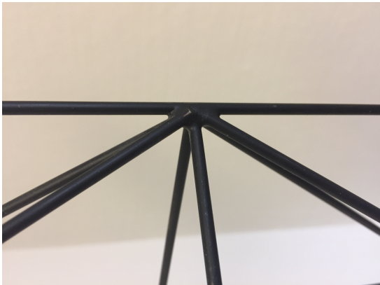
Figure 3.1: Shows the welded joint
