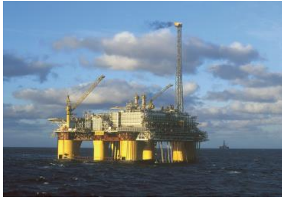
Figure2.13 (2): Åsgard B.production loop [4, p.2]. (Photo: Øyvind Hagen / StatoilHydro)
