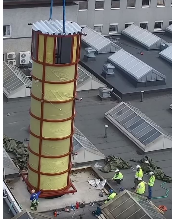
Figure 1.2: Installation of outer part of tower (Adressa)
