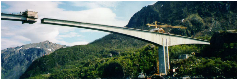
Figur 3.3: Snart sammenkobling [5]
