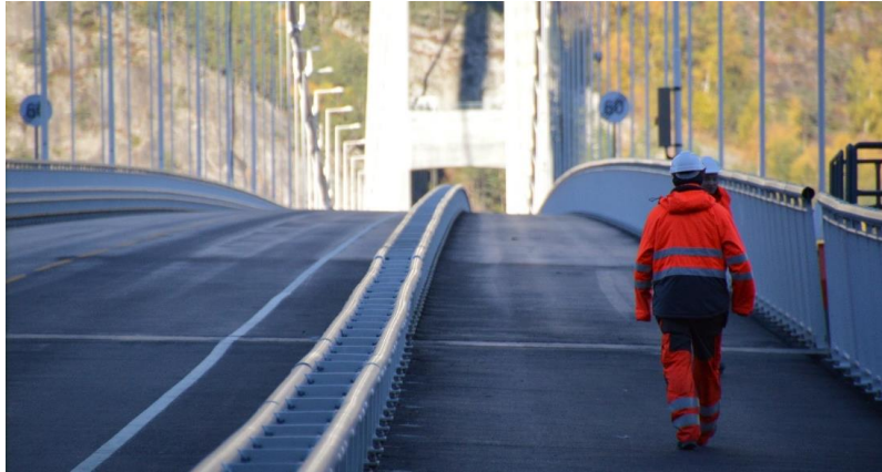
Fig. 6 On the deck of Hardanger Bridge: the curvature of the deck is visible
