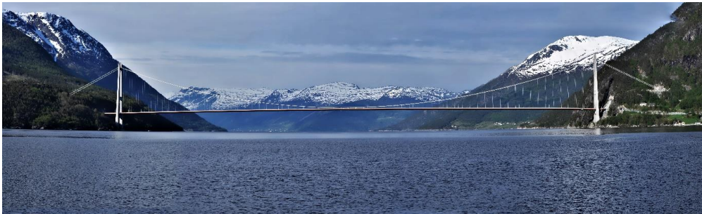
Fig. 3 Panorama view of the Hardanger Bridge. In the background, the tall mountains to the west can be observed. Mount Oksen stands on the right side i.e. the north end of the bridge, reaching up to 1000-1100 meters. (Photography by Aksel Fenerci/NTNU)
