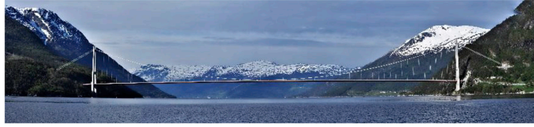
Fig. 1. Panoramic view of the Hardanger Bridge toward the west (photograph by Aksel Fenerci/NTNU).
