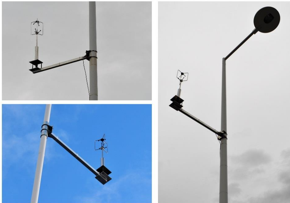
Fig. 9 Triaxial sonic anemometers installed on the Hardanger Bridge: the anemometers extend one meter to the side of the hangers by a steel bar to avoid disturbance of the wind flow. On the right, anemometer A6 is shown. It is attached to a light pole around midspan.
