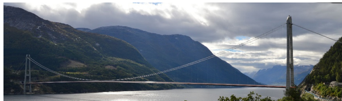
Fig. 1. The Hardanger Bridge.
