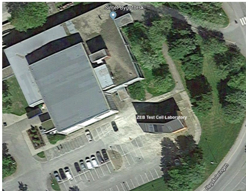
Figure 4.3.: Aerial photo of the ZEB Test Cell Laboratory and nearby surroundings, Ref.: ( Google Maps ).
