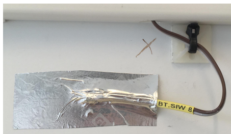
Figure A.2.: Thermocouple sensor measuring surface temperature.
