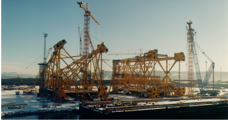
Figure 8.2: Assembled Steel Jackets at Aker Verdal
