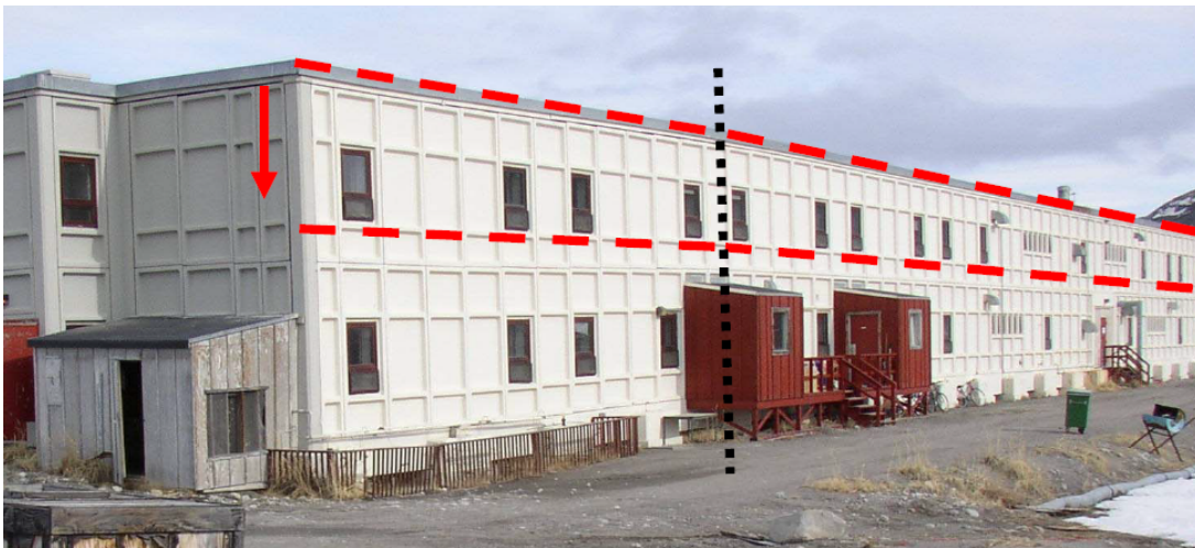
Figure 1.6: Uneven permafrost thawing underneath a building foundation in Kangerlussuaq (Ingeman-Nielsen, 2017); vulnerability to subsidence is widespread in the Arctic due to seasonally natural freeze-thaw cycles but it is expected to increase under conditions of global warming (Nelson et al., 2001)
