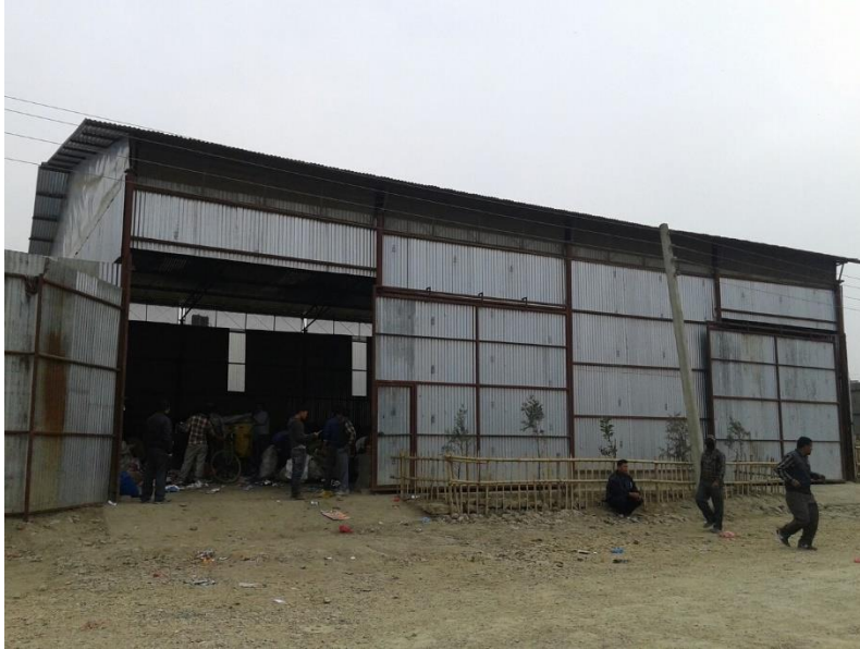
Figure 9: Transfer Station of an NGO.
