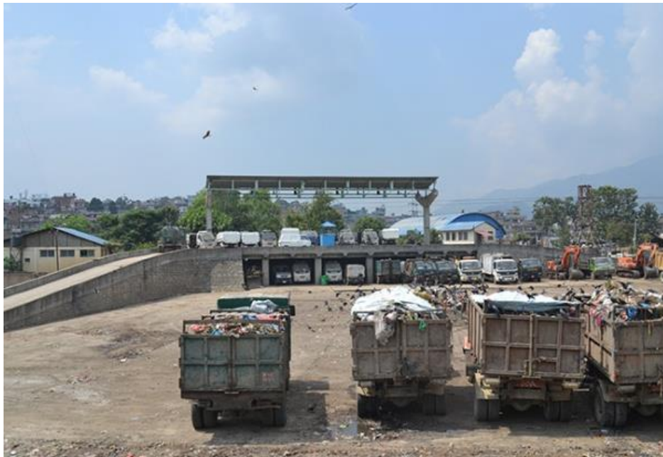
Figure 10: Municipal Transfer Station.
