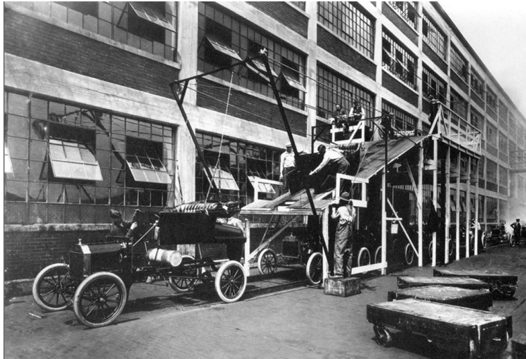
Figure 2.1: Ford Model T assembly line, 1913.
