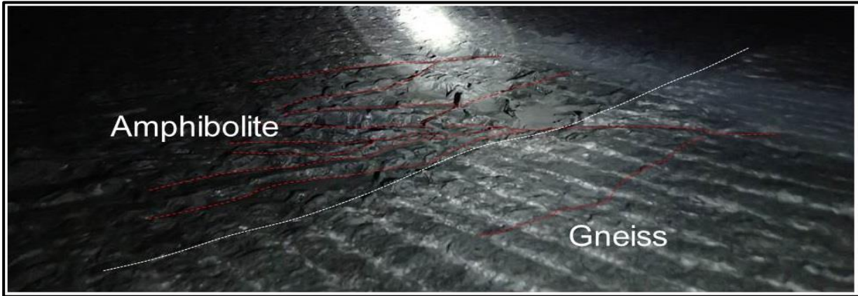
Figure 4.1 – Example of a face inspection with different rock types and degree of fracturing. Notice the high fracture frequency in the amphibolite (marked in red). Photo: Bane NOR (2018).
