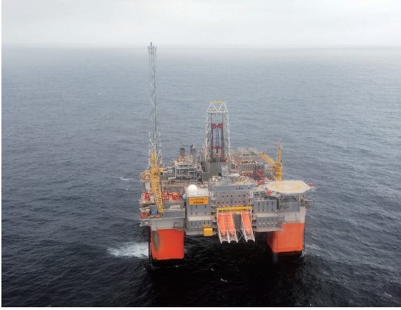
Fig. 1. Snorre B O&G platform in the Norwegian North Sea (photo: courtesy of Statoil).
