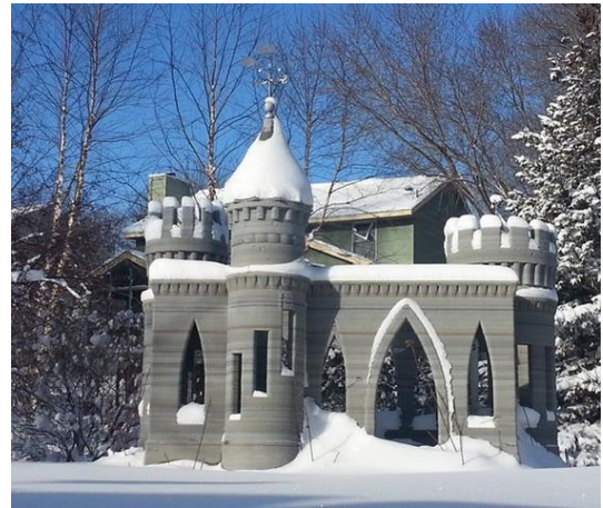
Fig. 2. Concrete Castle: This castle was built in cement in 2014 using Total Kustom's AM technology. This was their first large project, and the structure was therefore built piece by piece, and then assembled afterward. Photo: www.totalkustom.com [12].
