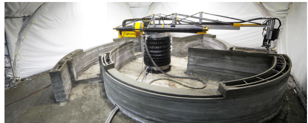
Fig. 3. Apis Cor House: The robot manipulator used in their project is similar to a tower crane, with a workspace in a circular area around its base. Photo: www.totalkustom.com [14].
