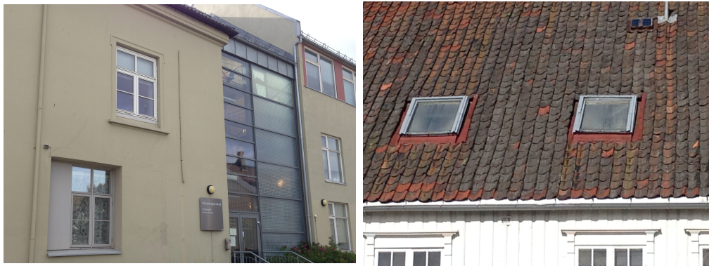
Figure 17: An original 1904 building with curtain walls as an extension connecting it to the neighbouring building (left) and old skylight windows in an original 1830 building (right)
