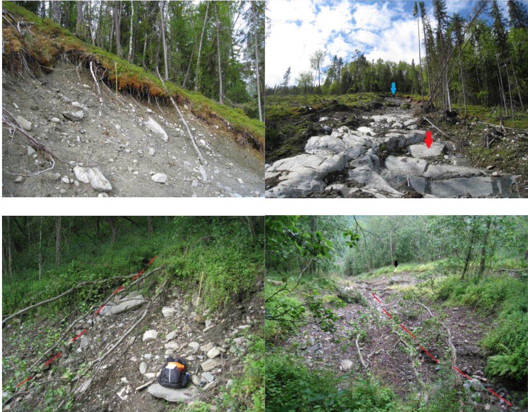
Figure 4.12: Top photos: Slide triggered on a clear-felled area south of the river in Kvam. Left: Triggering zone. Right: Same landslide seen from below. Blue arrow indicates the triggering zone and red arrow points to exposed bedrock in the slide path. Bottom photos: Slide triggered in forested hill side of Veikledalen. Left: Trigger zone. Right: Same slide path seen standing in the triggering zone. Photos by: Edvardsen (2013), included with permission.
