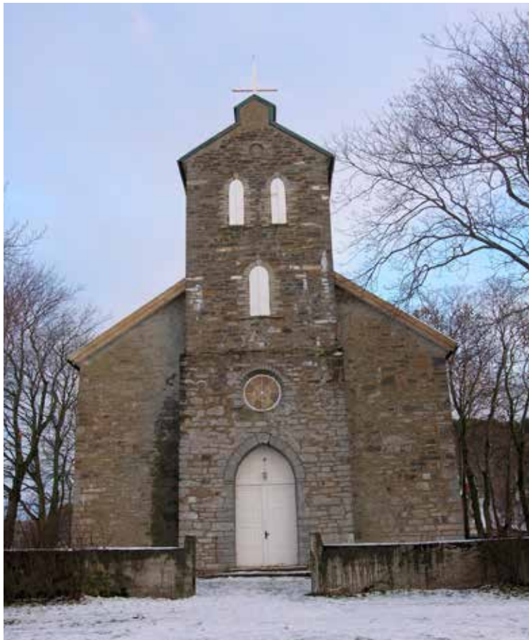
Figure 6. The west front of Tjøtta church as it appears today after the last rebuilding finished in 1851. Soapstone ashlars from the medieval church are visible in the wall together with rubble stone. (Photo: B. Berglund).
