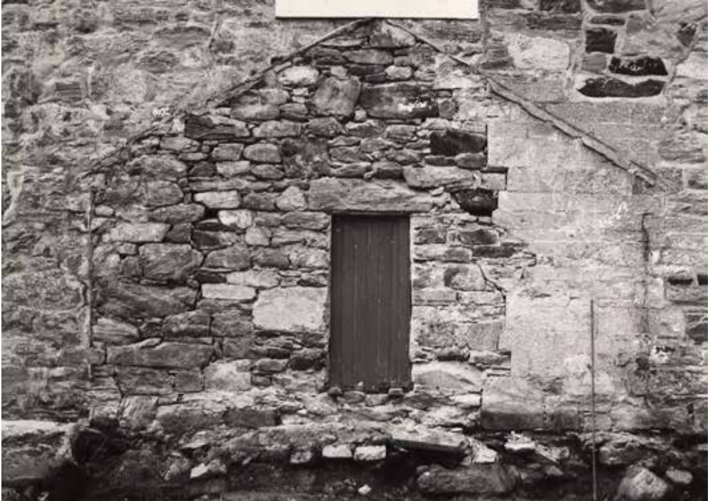
Figure 8. The outer east wall of the chancel in Brønnøy church. The photograph from 1960 shows that a section of the medieval wall with soapstone ashlars is preserved. (Photo: E. Høvding. ©The Directorate for Cultural Heritage, The Archive).
