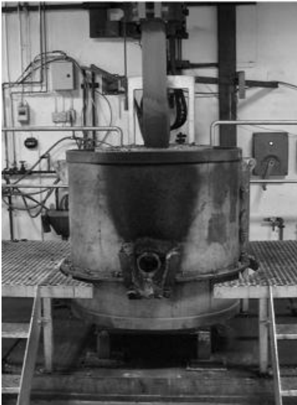
Figure 6-1: Picture of the 150 kVA one phase furnace (Slizovskiy et al. 2007).
