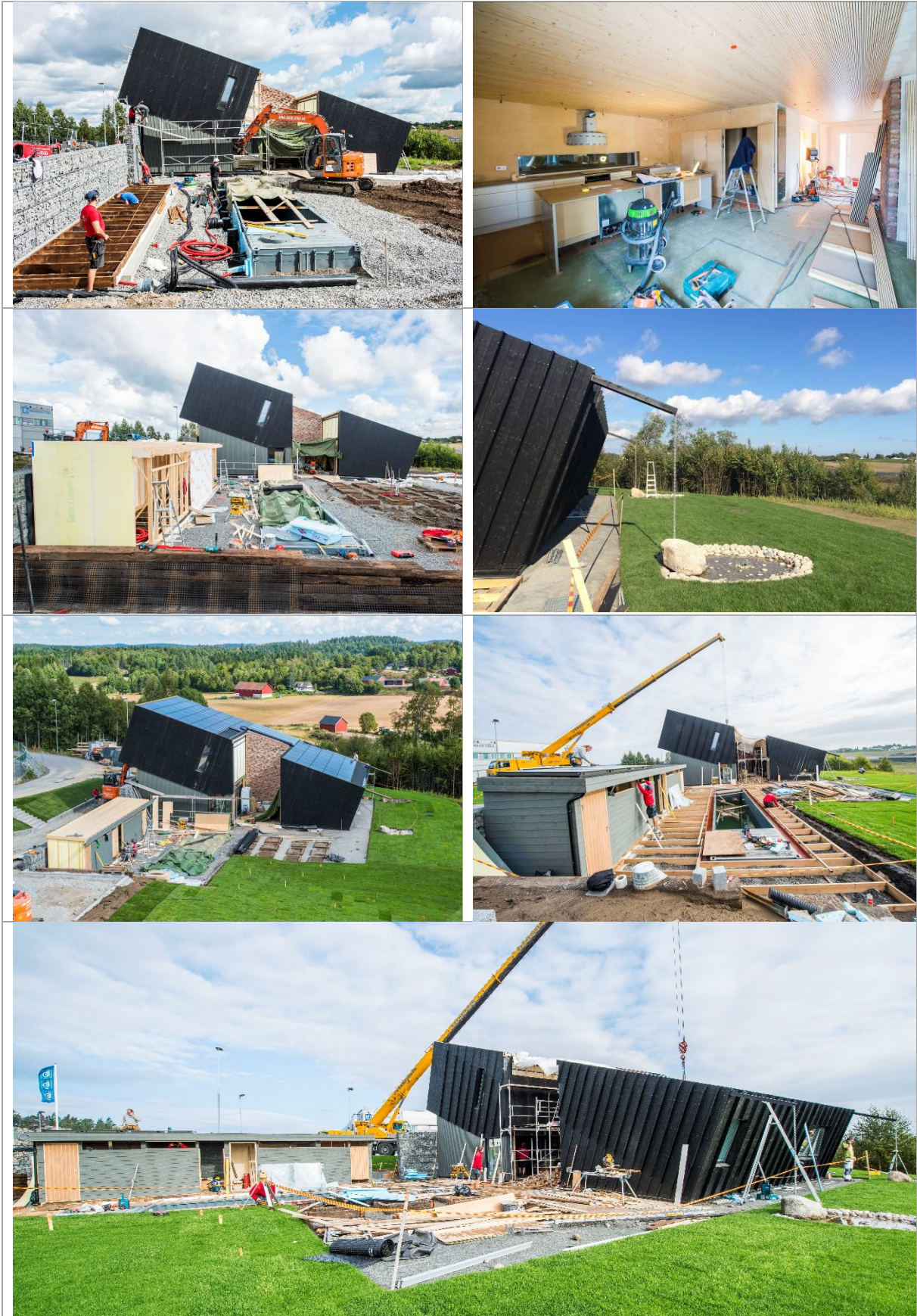
Figure 9.2 Pictures from the construction process (photos: Brødrene Dahl/Paal-André Schwital).
