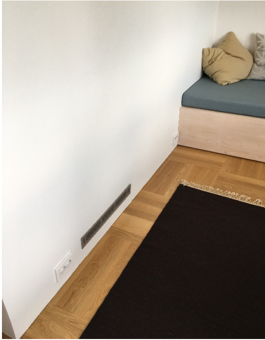
Figure 3.2 Ventilation grilles in the house (photo: SINTEF)
