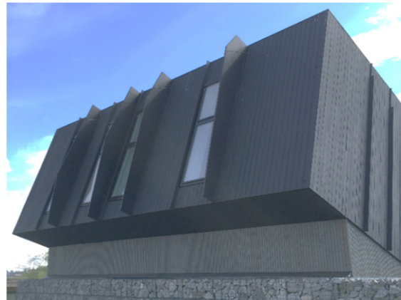
Figure 2.9 Solar protection on the bedroom windows. Photo: SINTEF Byggforsk.
