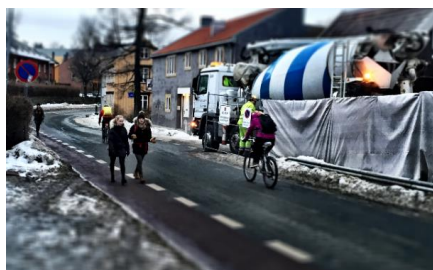
Figure 33 – Construction site in city centre affecting the adjacent cycle lane, Trondheim
