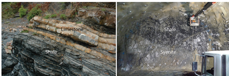
Fig. 3: Alternating shale and limestone layers of stage 3a (left) from Nærnes southwest of Oslo. Photo: Kjetil Lenes (CC BY-SA 3.0). Syenite intrusion and shale of probably stage 4b exposed in the Løren road tunnel (right) north of the city center. Pregrouting can be seen ongoing. Photo: From Høien and Nilsen (2014)
