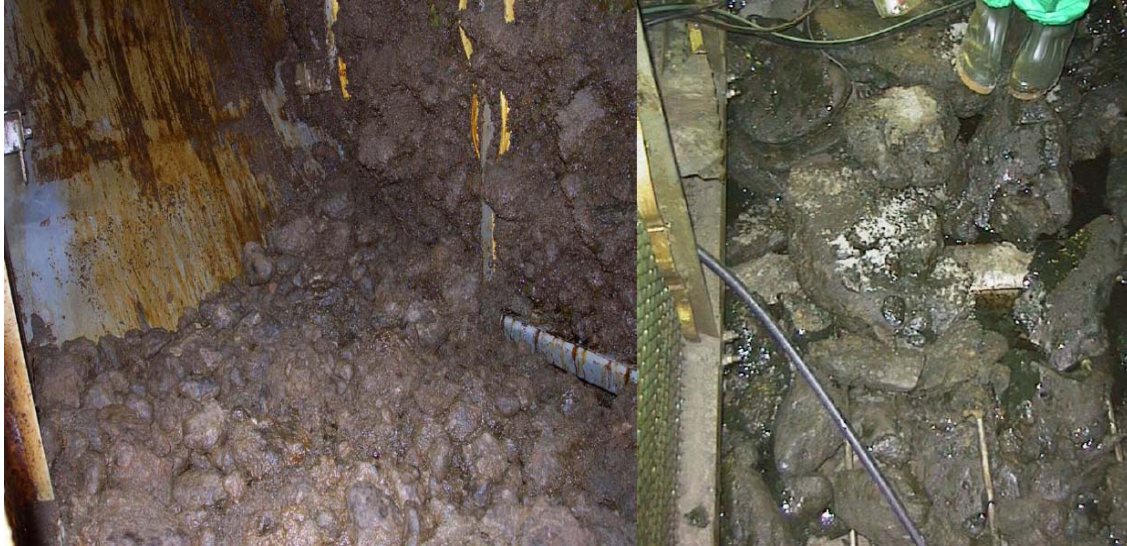
Figure 1.11: Calcium naphthenate build-up in separator [29].
