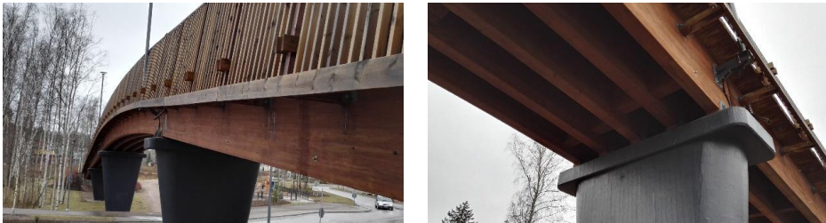
Fig. 2.1 Beam footbridge in Helsinki, Finland. Photo: A.W. Ostrycharczyk.
