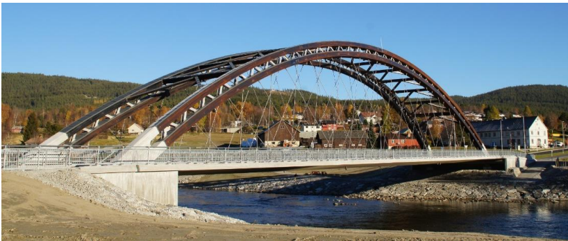
Fig. 3.18 Steien bridge, Norway – view of the network. Photo: Norwegian Public Roads Administration.
