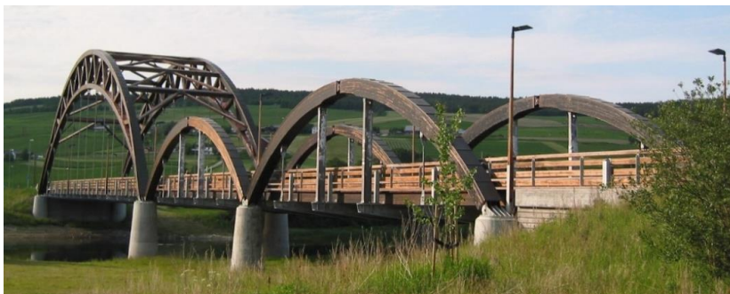
Fig. 2.7 Tynset bridge, Norway. Photo: K. Bell.
