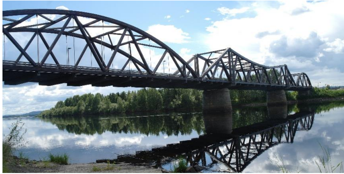
Fig. 2.4 Flisa bridge, Norway. Photo: M. Čepelka.
