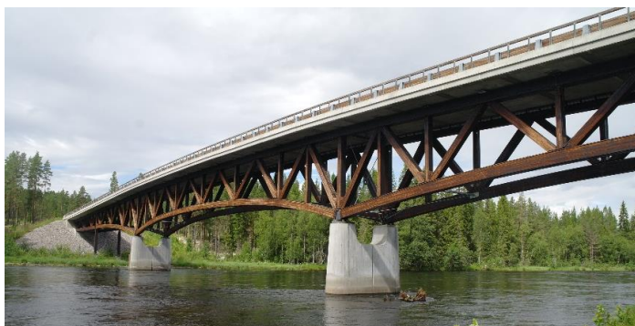
Fig. 2.3 Kjølssæter bridge in Åmot, Norway. Photo: M. Čepelka.
