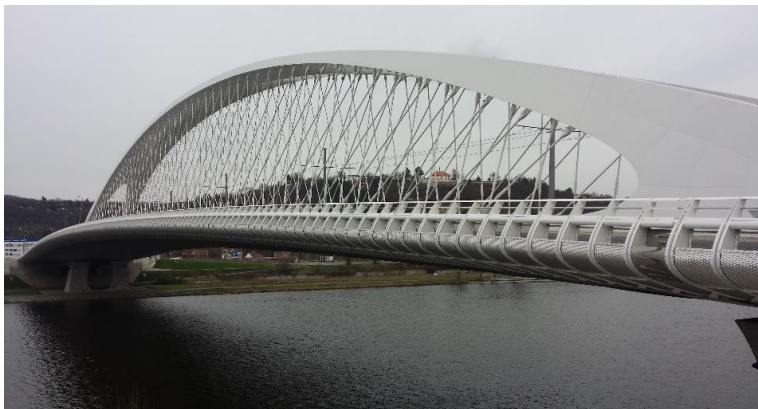
Fig. 3.20 Troja Bridge, Prague, Czech Republic. Photo: M. Čepelka.
