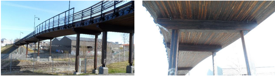
Fig. 2.2 Dalen slab footbridge in Trondheim, Norway. Photo: A.W. Ostrycharczyk.
