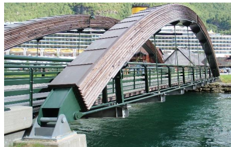
Fig. 3.2 Fretheim Bridge. Photo: Norwegian Public Roads Administration.
