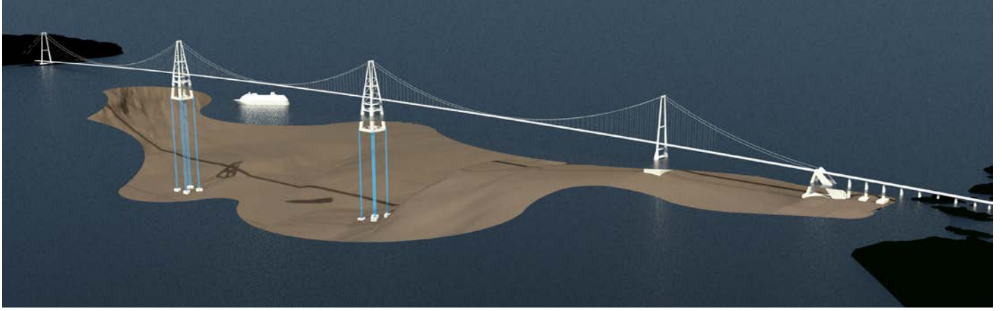
FIGURE 1. A THREE-SPAN SUSPENSION BRIDGE WITH TWO FLOATING PYLONS. ILLUSTRATED BY ARNE JØRGEN MYHRE, STATENS VEGVESEN
