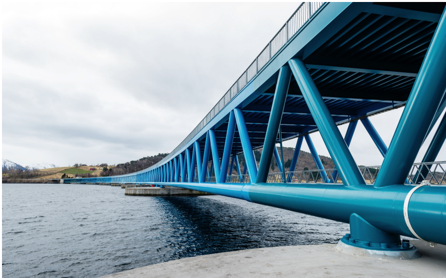
Figure 1: The Bergsøysund Bridge. Photograph by NTNU/K. A. Kvåle.
