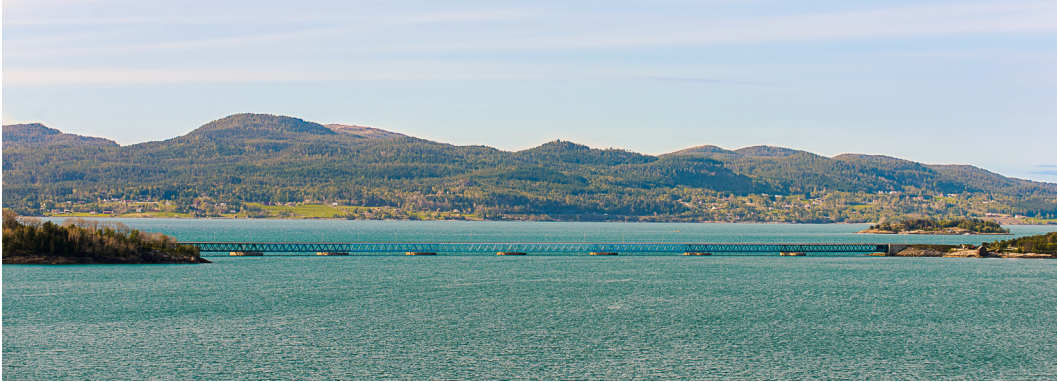
Fig. 1: The Bergsøysund Bridge. Photograph by NTNU/K. A. Kvåle.
