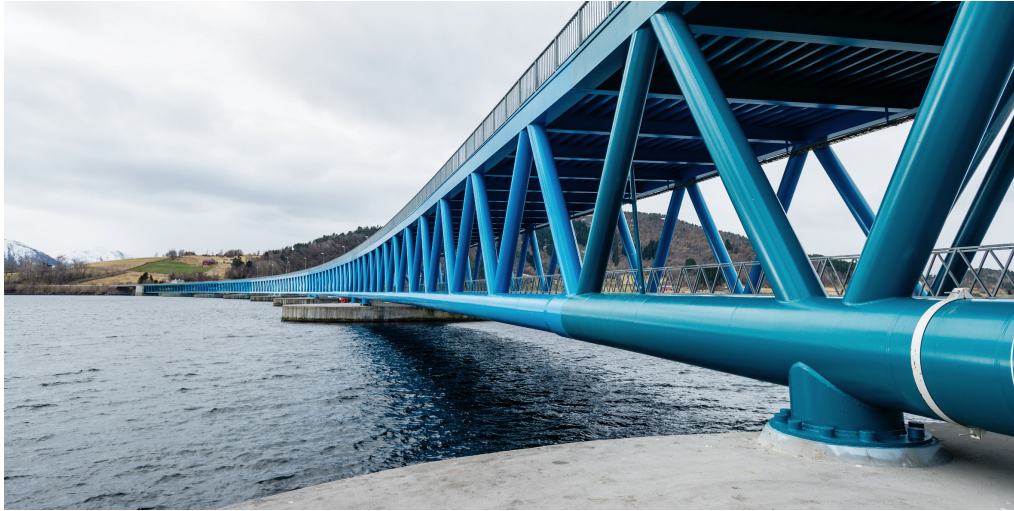
Figure 1. The Bergsøysund Bridge. Photograph by NTNU/K.A. Kvåle.
