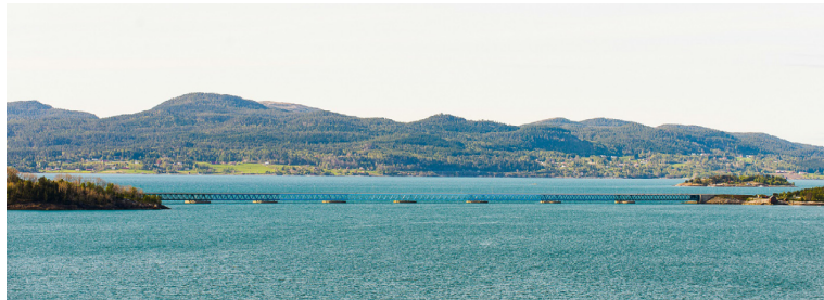
Fig. 2. The Bergsøysund Bridge. Photograph by NTNU/K.A. Kvåle.
