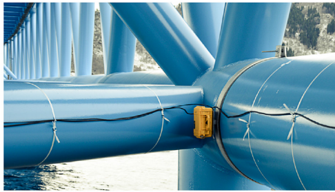
(a) CSI CUSP-3 accelerometer on truss. Closed protection box.
