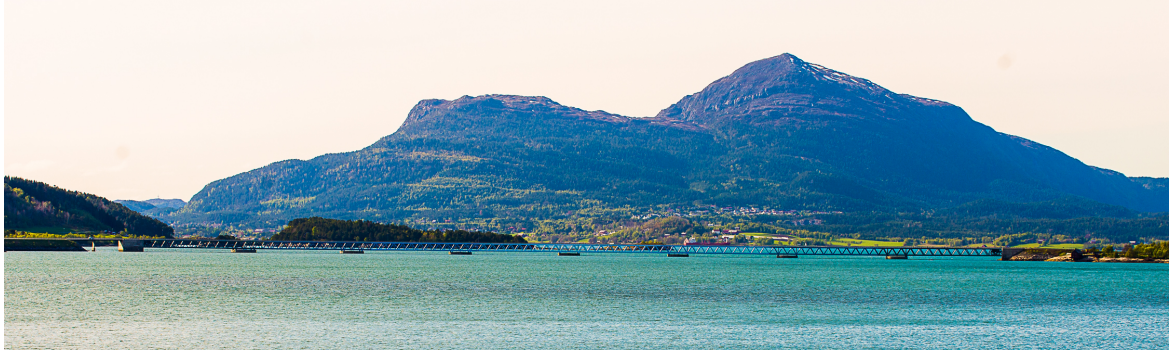
Fig. 1. Photograph of the Bergsøysund Bridge. Photograph by NTNU/K.A. Kvåle.
