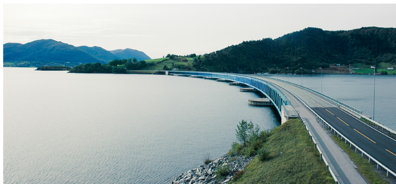
Fig. 1. The Bergsøysund Bridge. Photograph by NTNU/K.A. Kvåle.
