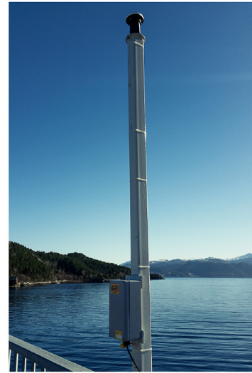
(e) Trimble RTK GNSS sensor in designated pole.
