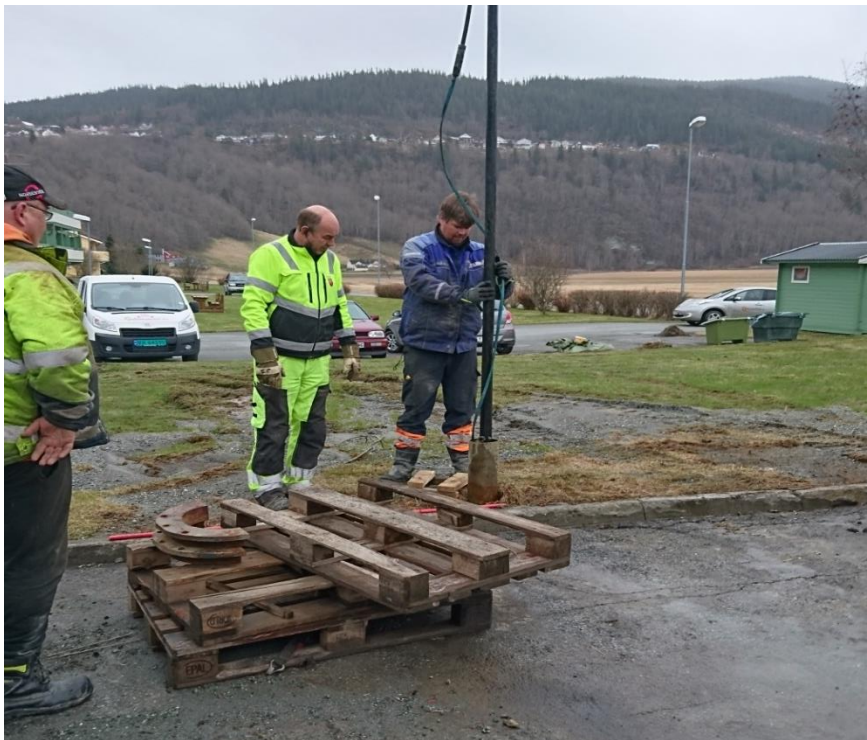
Figure 16: Well at fire station in Melhus (Source: NGU database)
