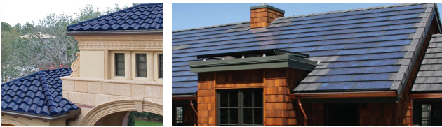
Fig.1. Examples of BIPV tiles on building roofs, Solar Thermal Magazine (left) [1] and Applied Solar (right) [2].
