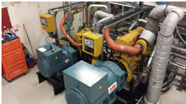
FIGURE 8. Diesel generators of the HML at NTNU, courtesy: ABB.
