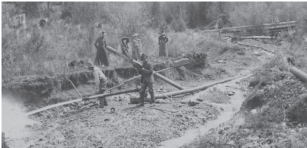
Figure 2.1. A small, hydraulic gold mining operation in what was then Oregon Territory, from 1885, at the northwestern coast of today's U.S.A. ( http://www.miningartifacts.org/ ).
