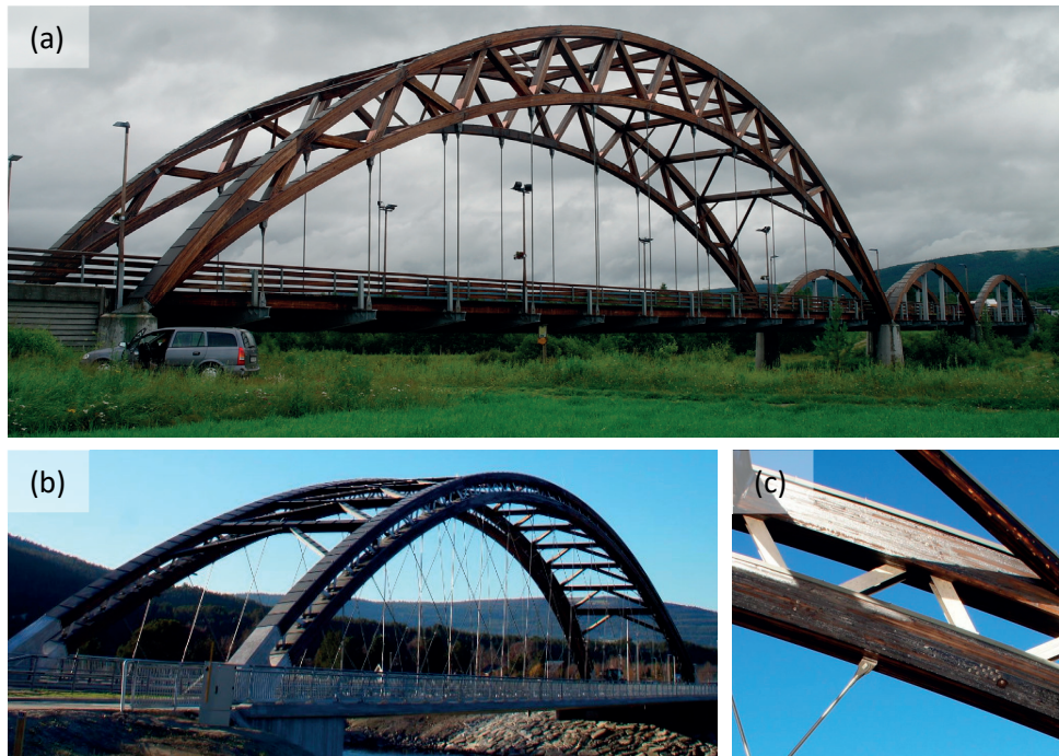
Figure 1.1 Large road timber arch bridges in Norway: (a) the Tynset Bridge (2001), (b) the Steien Bridge (2016) [3], (c) detail of the arch of the Steien Bridge [3]
