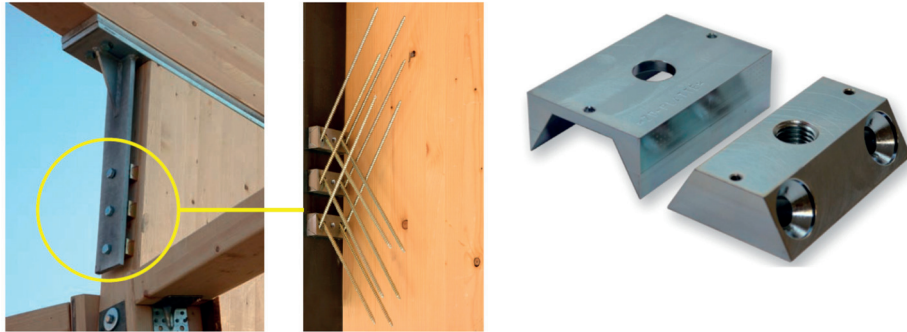
Figure 2.13 Joint with ZD-plates and STS screws [63]: portal frame joint (left), detail of screw assembly (centre), ZD-plate (right)
