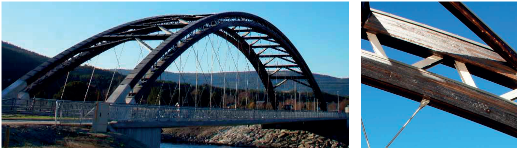
Figure 1: Steibrua, Norway – Network arch bridge with glulam arches [6].
