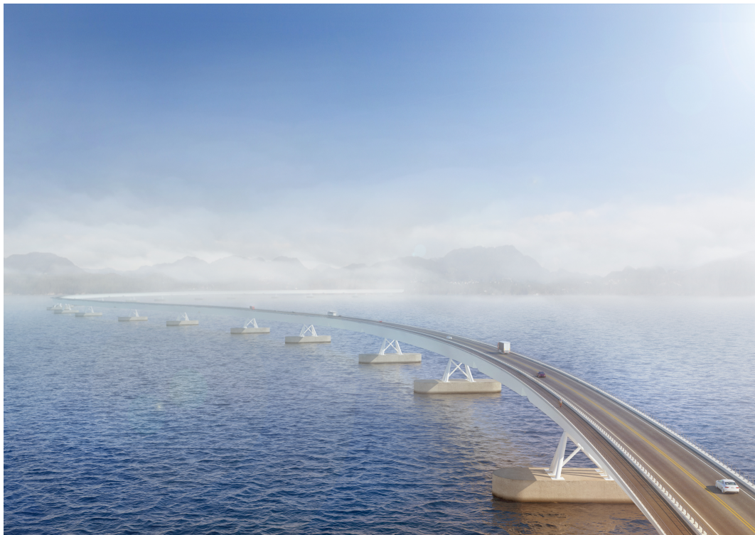
Figure 11: Chained floating bridge, illustration by Multiconsult.
