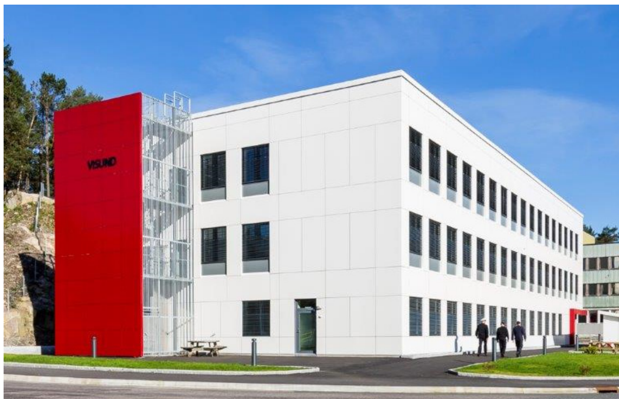
Figure 1.1 The south (long) and west (short) façade of the building. Photo: Forsvarsbygg / Hundven-Clements Photography.
