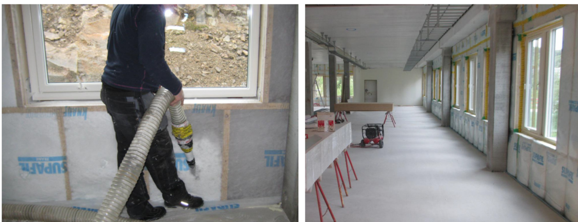
Figure 7.2 Thermal insulation on external walls. Photo: Forsvarsbygg.
