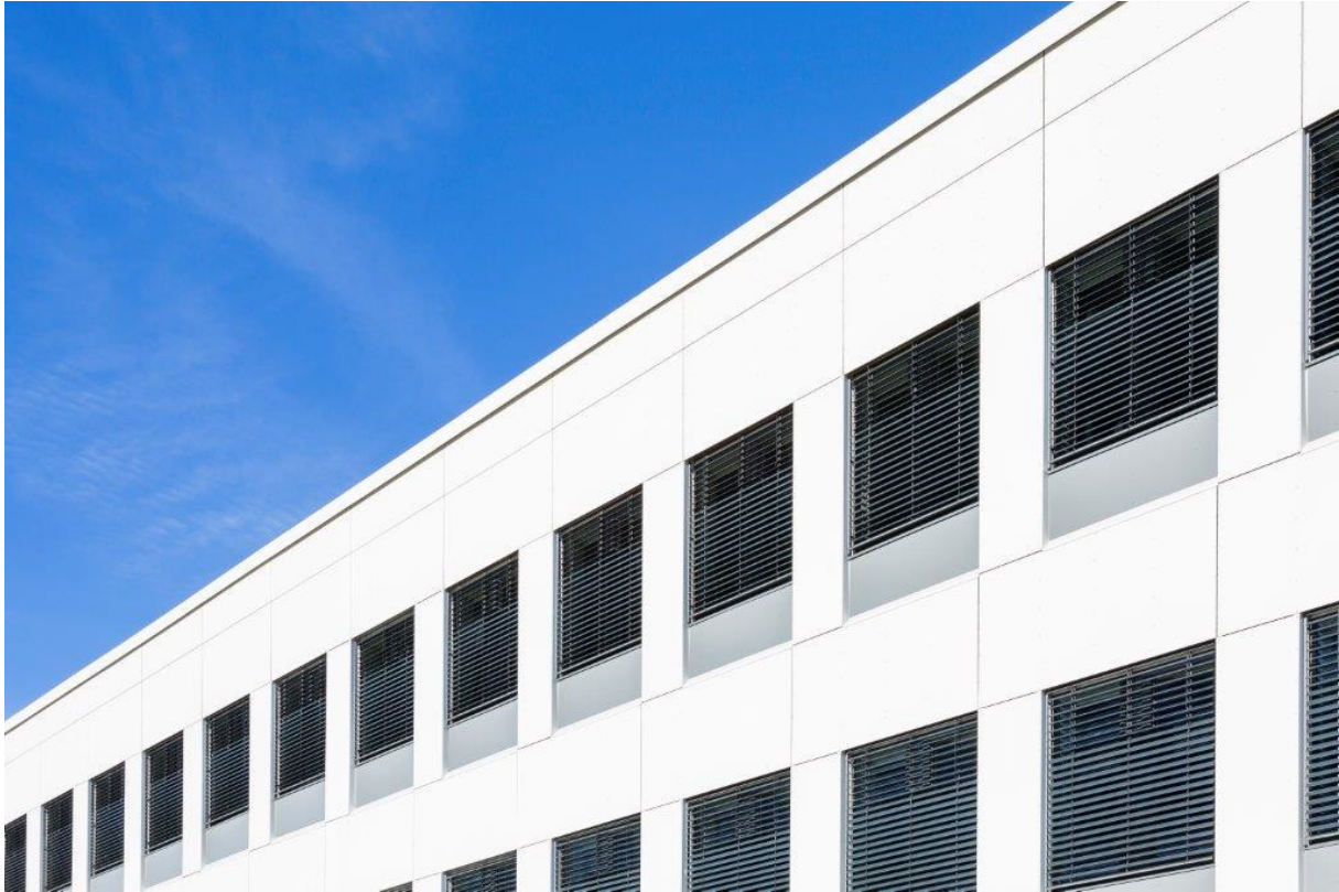
Figure 3.4 The exterior sun shading system. Photo: Forsvarsbygg / Hundven-Clements Photography.
