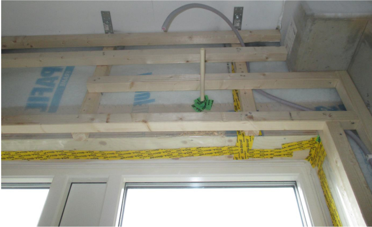
Figure 7.3 Building of air tight walls. Photo: Forsvarsbygg.
