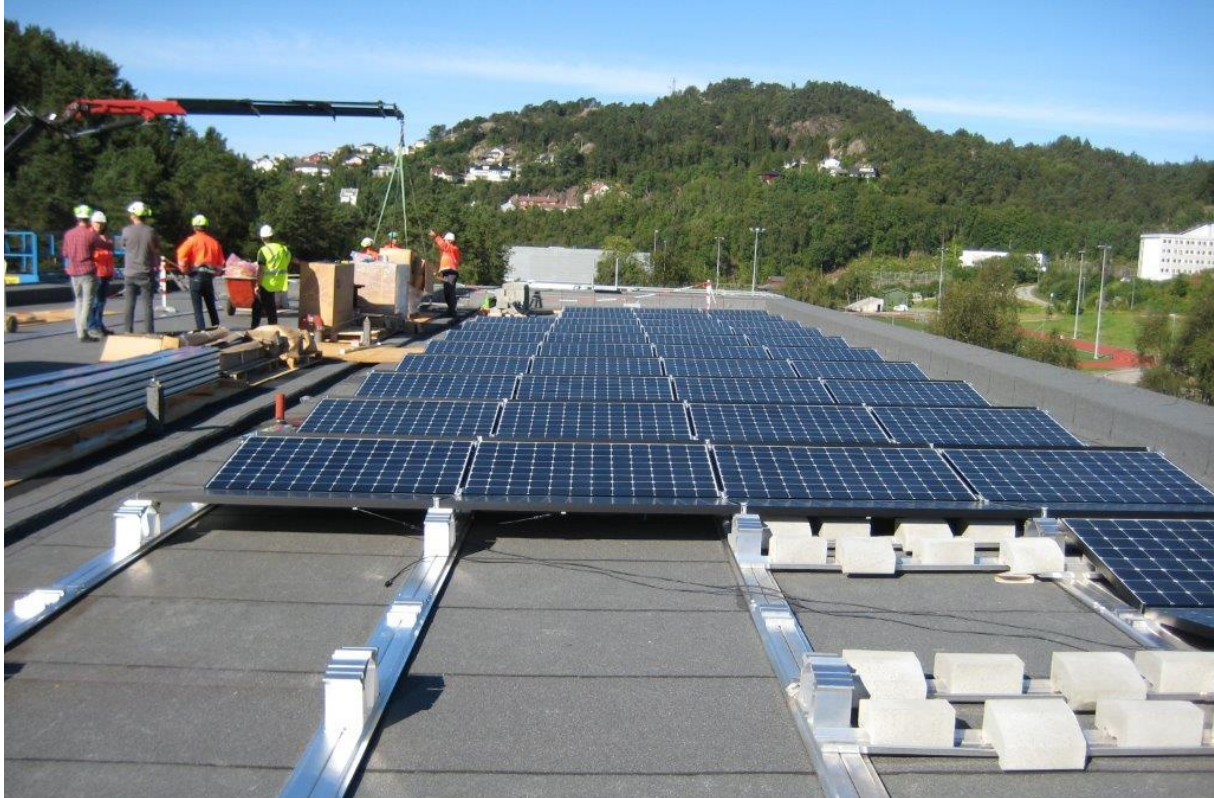
Figure 4.3 The installation of the PV panels on the roof. Source: Veidekke.
