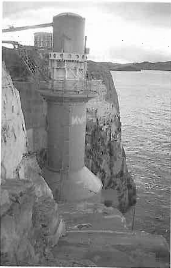
Figure 7. The Kvaerner OWC wave power plant constructed in a steep shore cliff at Toftestallen.
