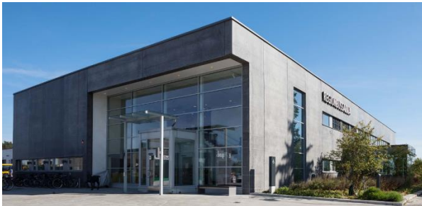
The Building entrance to Fyrislund bus depot.
