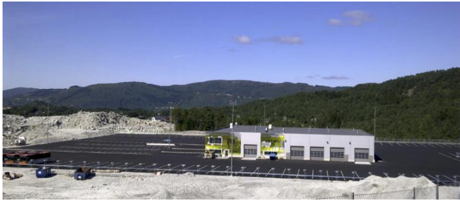
Figure 4.22 Bus depot Haukås. Source: Department of Real Estate, Hordaland County.
