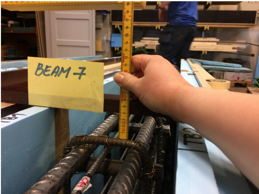
Figure A.22: Beam 7 - Concrete cover
