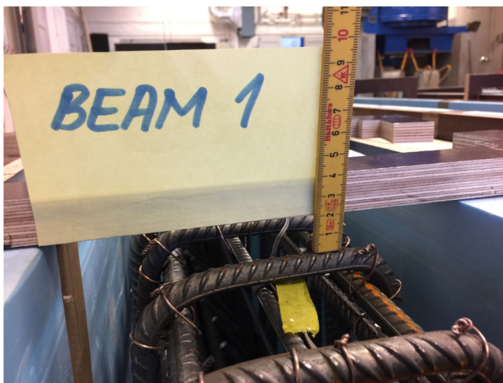
Figure A.10: Beam 1 - Concrete cover
