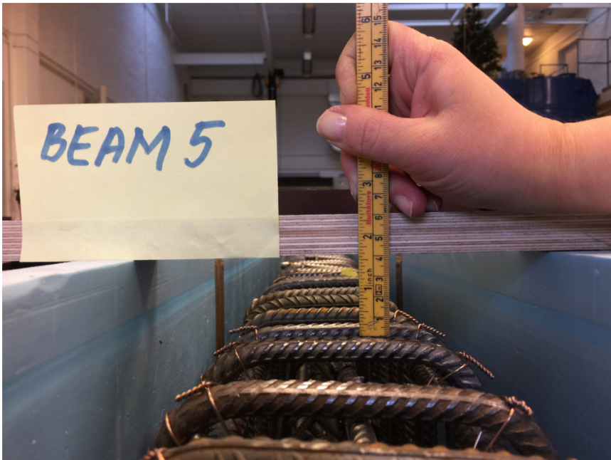
Figure A.18: Beam 5 - Concrete cover
