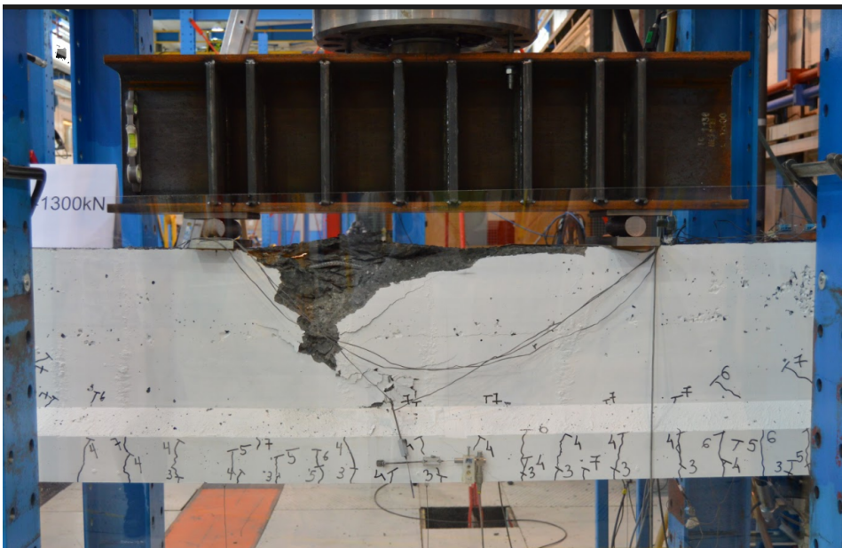
Figure 5.23: Beam 2 - Test zone, failure
